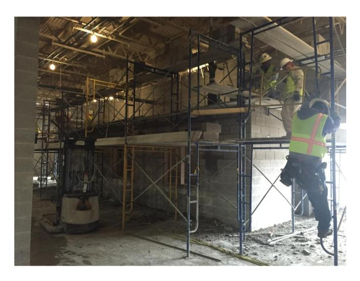
**INTERIOR WALLS** – Non-Load bearing concrete block interior walls are being erected at the gymnasiums. The structural steel has been fireproofed.
